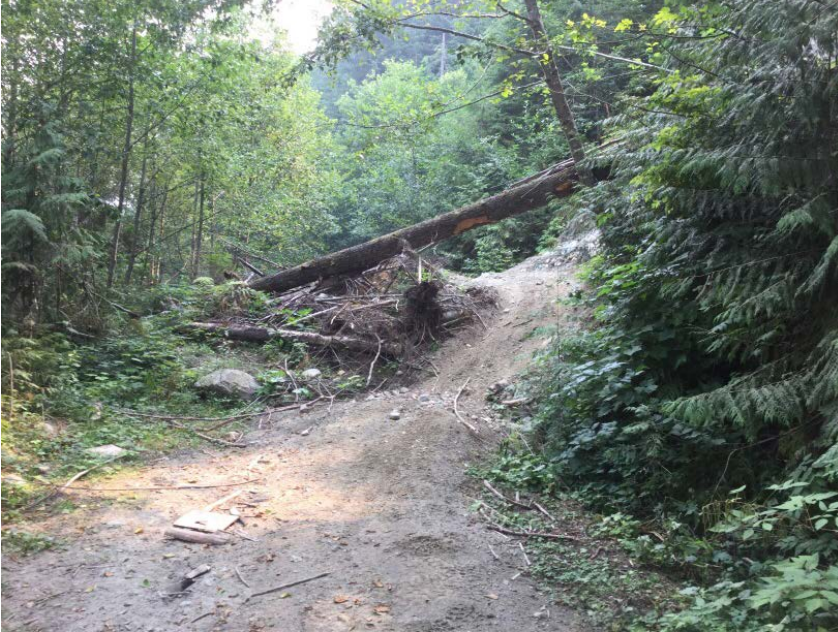
Road blocked at this location, only passable to Off Road Vehicles
